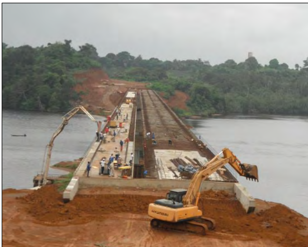
Figure 4-2 Mayumba Bridge (SRK, 10 January 2014)
