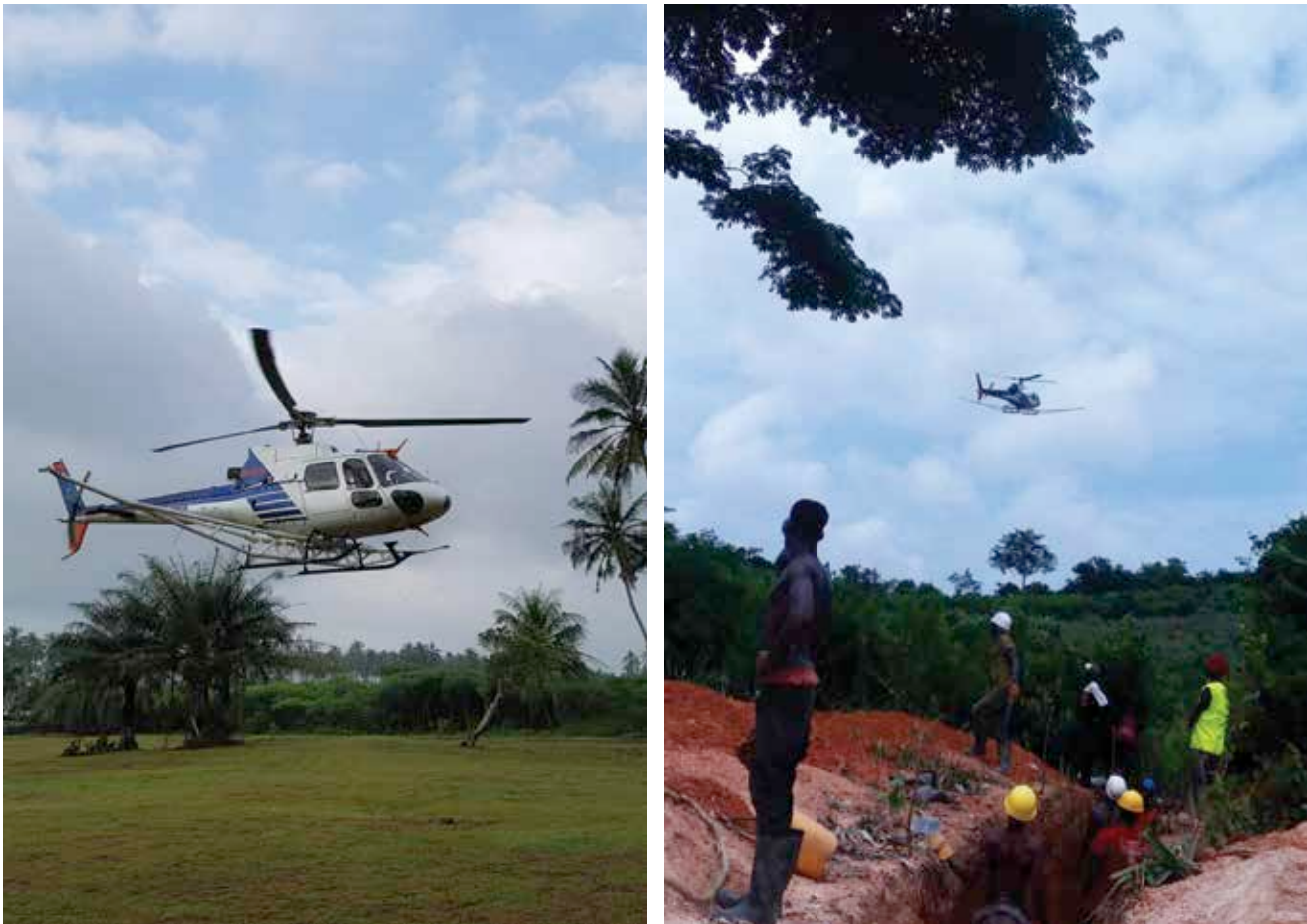
Figure 8: (LEFT) New Resolution Geophysics (NRG) helicopter with geophysical equipment taking off from Cape Coast base and (RIGHT) trenching underway at the Ewoyaa prospect with light coloured spodumene bearing pegmatite in the trench.
